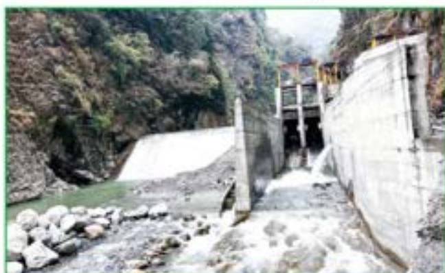
Headworks, viewing upstream
