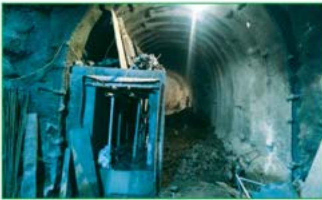
Sediment Flushing during construction
