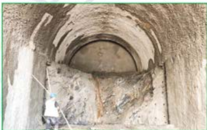
Tunnel Boring Machine-Platform Area-Entry Point
