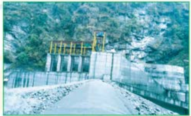
Hoisting system installation at undersluice and intake
