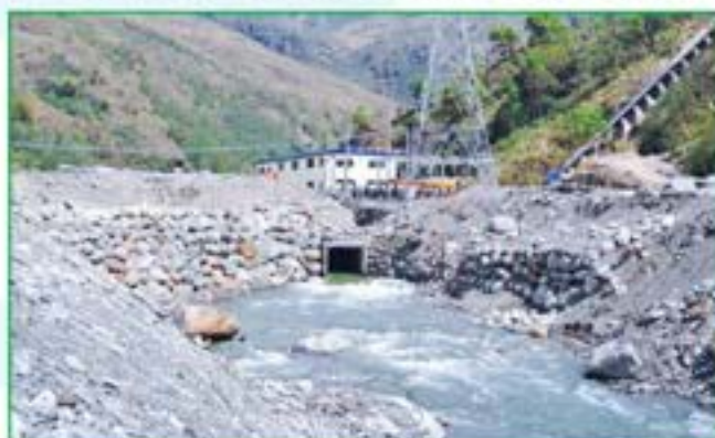
Outlet of tailrace culvert
