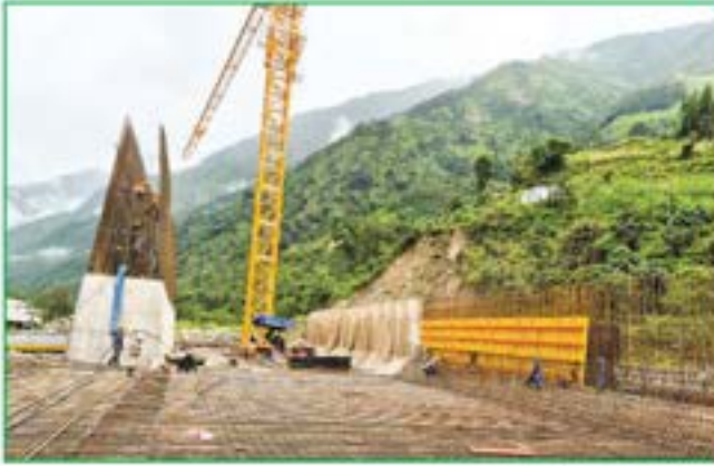
Construction of Settling Basin at Headworks
