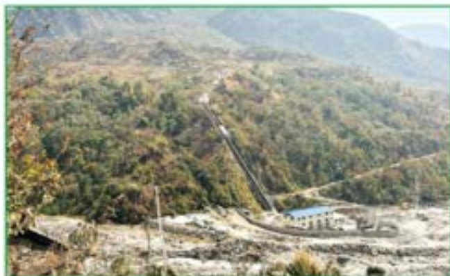
Overall view of penstock alignment
