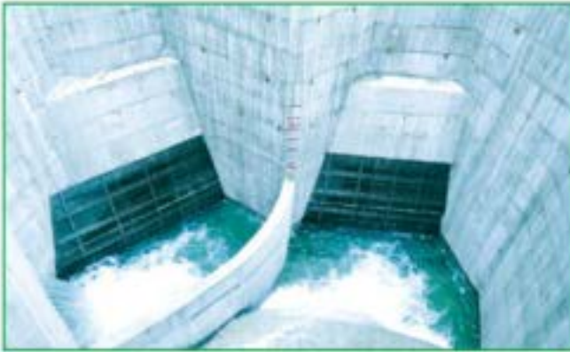
Water filling at intake/gravel trap
