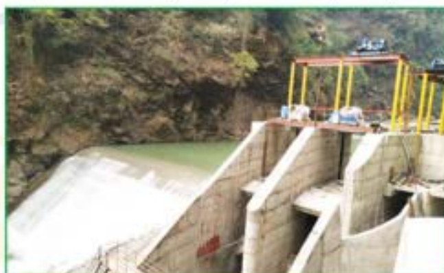
Water spilling through weir during wet test
