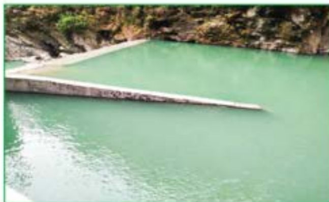
Upstream of weir, after operation of power plant
