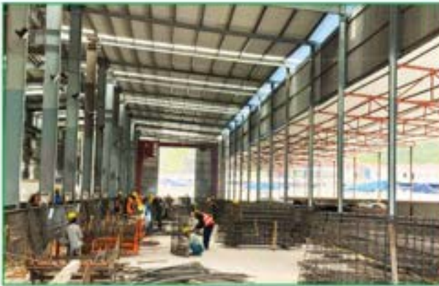
Reinforcement Cage for Segment Production
