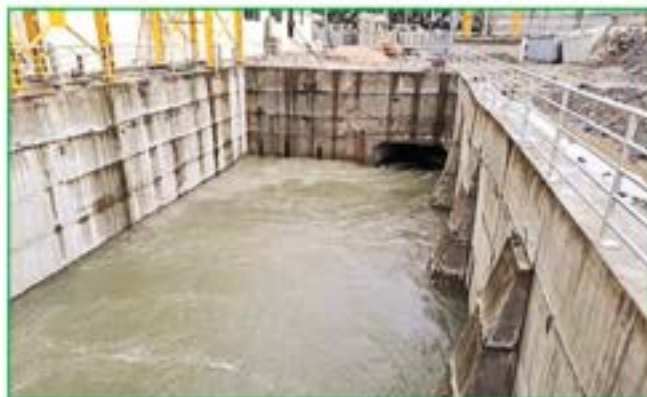
Tailrace Cooling Pool
