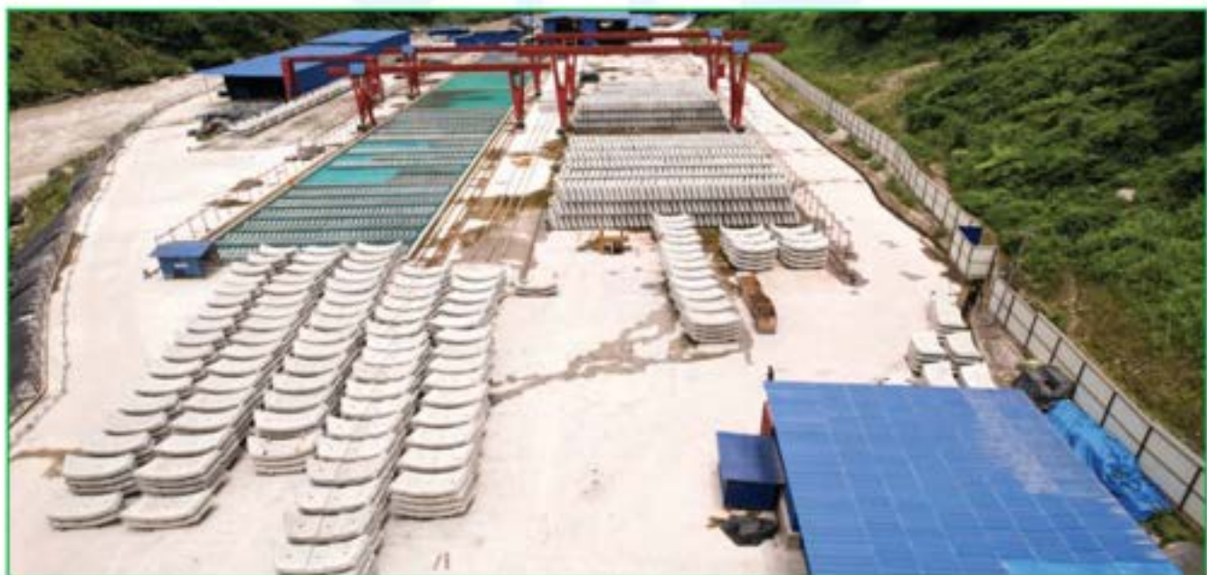
Segment Production Yard
