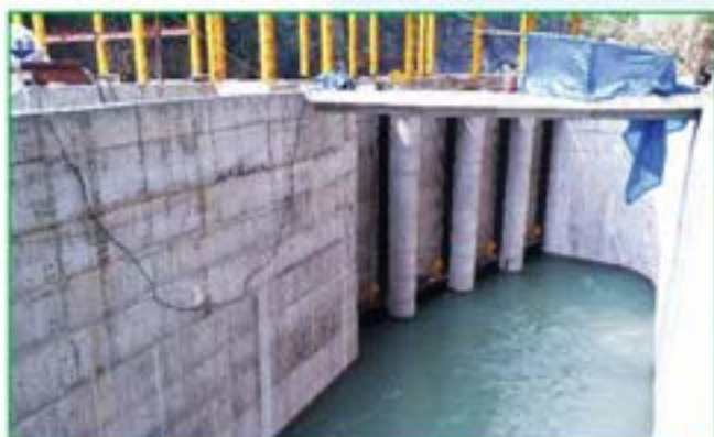
Water filling at intake/gravel trap.
